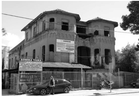
Fig. 1. The “Haunted House”, main front.
