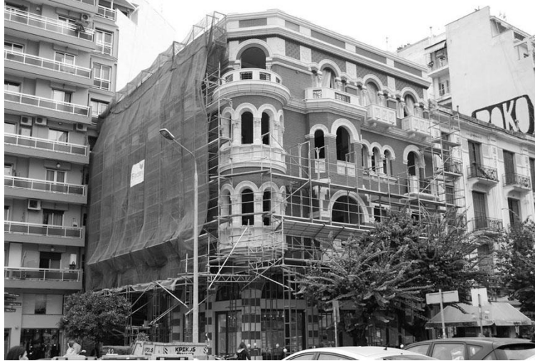
Fig. 7. The “Longos Mansion”, main front, under restoration.
