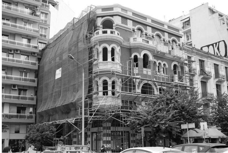
Fig. 7. The “Longos Mansion”, main front, under restoration.
