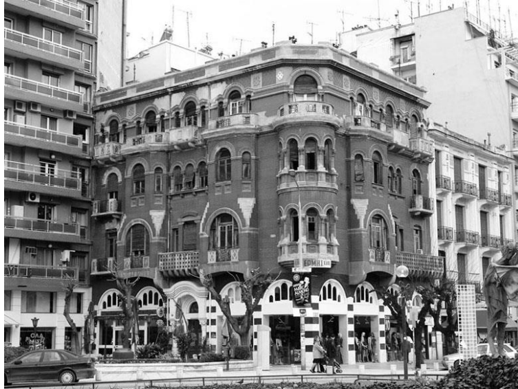
Fig. 5. The “Longos Mansion”, main front, prior to restoration.
