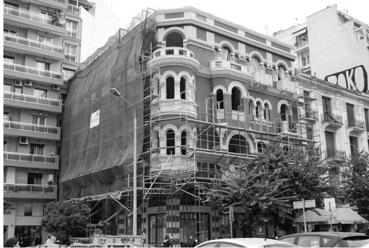
Fig. 7. The “Longos Mansion”, main front, under restoration.
