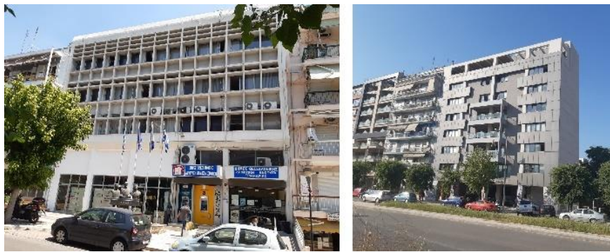
Fig. 1. The two case-study buildings. Left: Building A. Right: Building B.
