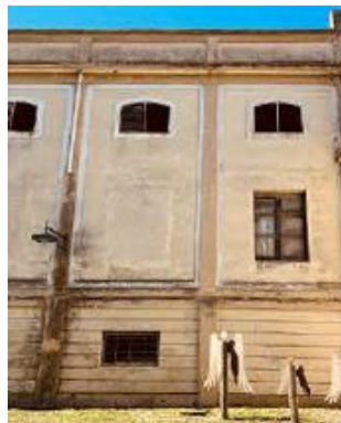
Fig. 7. Alternation of masonry walls and pillars on the façade
