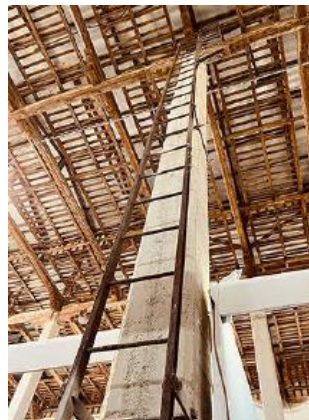
Fig. 8. Reinforced concrete pillar
