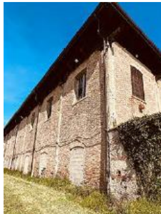
Fig. 10. Closure of the opening at ground floor
