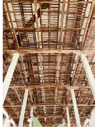
Fig. 9. The structure of the roof
