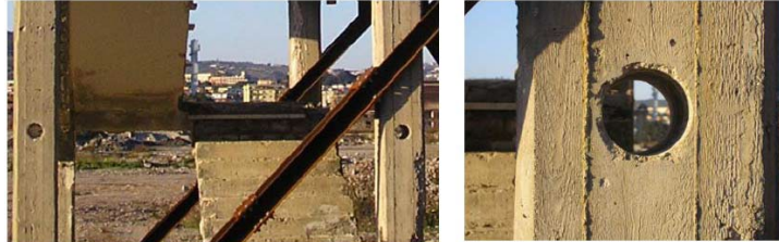
Fig. 10. Extraction of cylindrical cores from module n.6.
