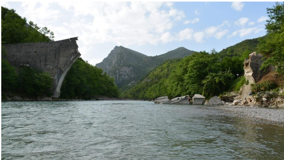
Fig. 2. Plaka Bridge (downstream view), May 2015.(Image source: © Ch. Giannelos)
