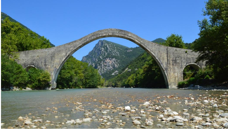
Fig. 1. Plaka Bridge (downstream view), August 2014.
