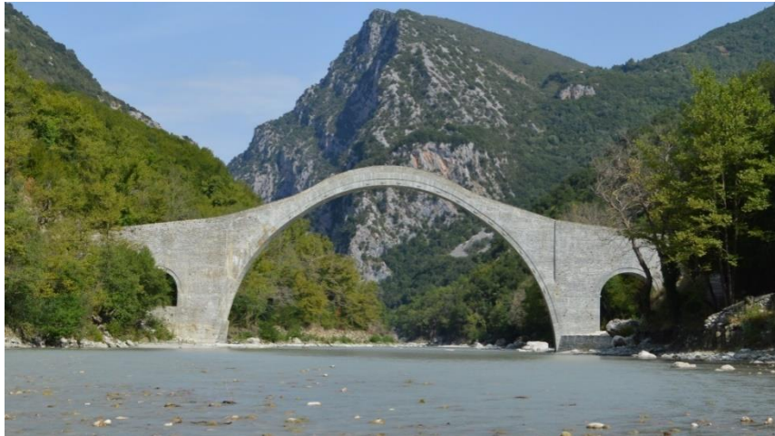
Fig.11. Plaka Bridge after restoration (downstream view), August 2021.
