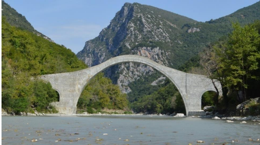
Fig.11. Plaka Bridge after restoration (downstream view), August 2021.
