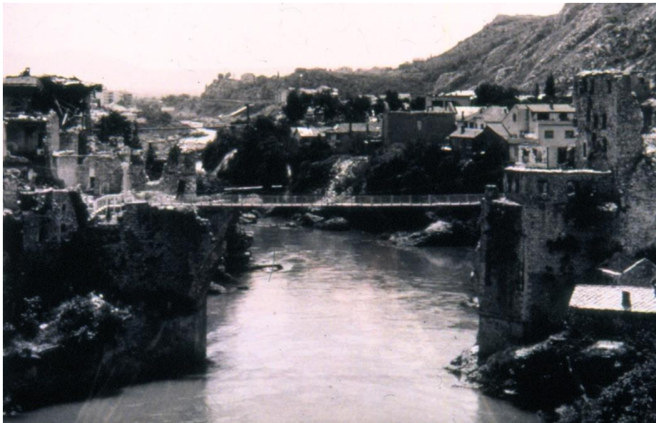
Fig.7. View of the temporary suspension bridge, February 1995.(Image source: © A. Pašić)
