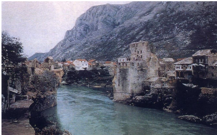
Fig. 4. The surviving abutments of Stari Most after the bombardment, December 1993. (Image source: © A. Pašić)
