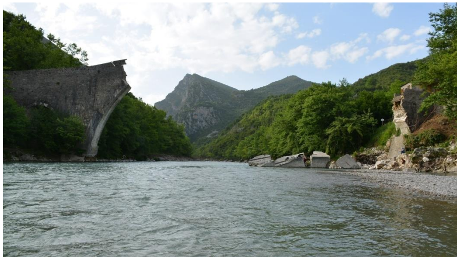
Fig. 2. Plaka Bridge (downstream view), May 2015.(Image source: © Ch. Giannelos)
