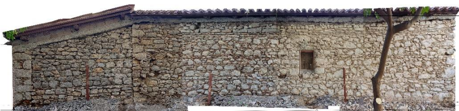
Fig. 12. Orthoimage of the south façade.
