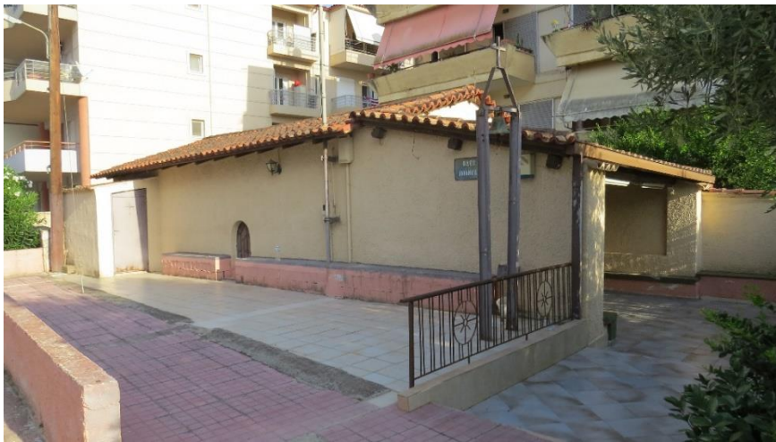
Fig. 1. North–West view of the church before the building works. (7/9/2021)
