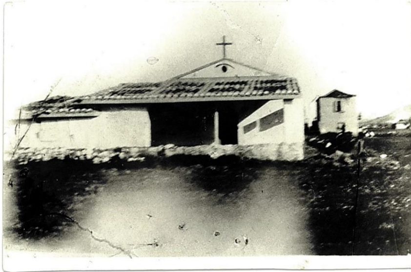
Fig.8. Photographic documentation of the west façade (adopted from [14]).
