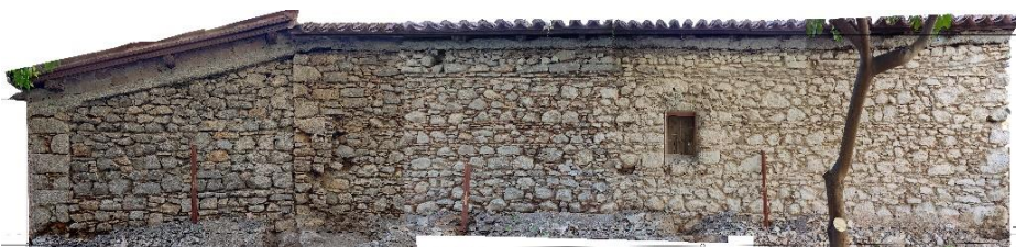
Fig. 12. Orthoimage of the south façade.
