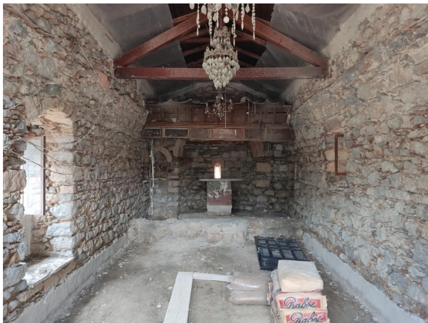
Fig. 5. Interior. Removal of plaster on the interior masonry. (23/6/2023)
