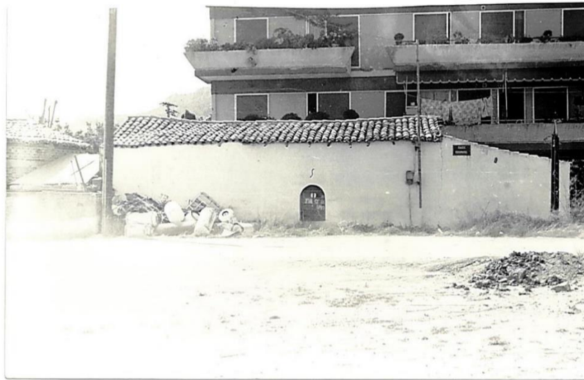
Fig.10. Photographic documentation of north facade (Adopted from [14]).
