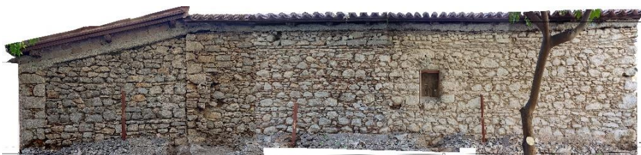
Fig. 12. Orthoimage of the south façade.
