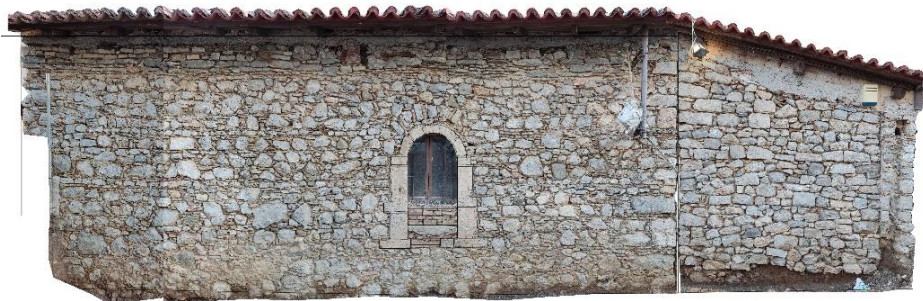
Fig. 11. Orthoimage of the north façade.
