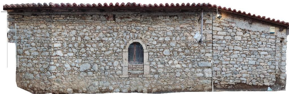
Fig. 11. Orthoimage of the north façade.
