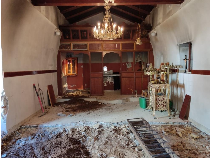
Fig. 4. Interior of the church. Test cuts on the interior masonry. Removal of interior floors Detachment of the newest part of the iconostasis.
