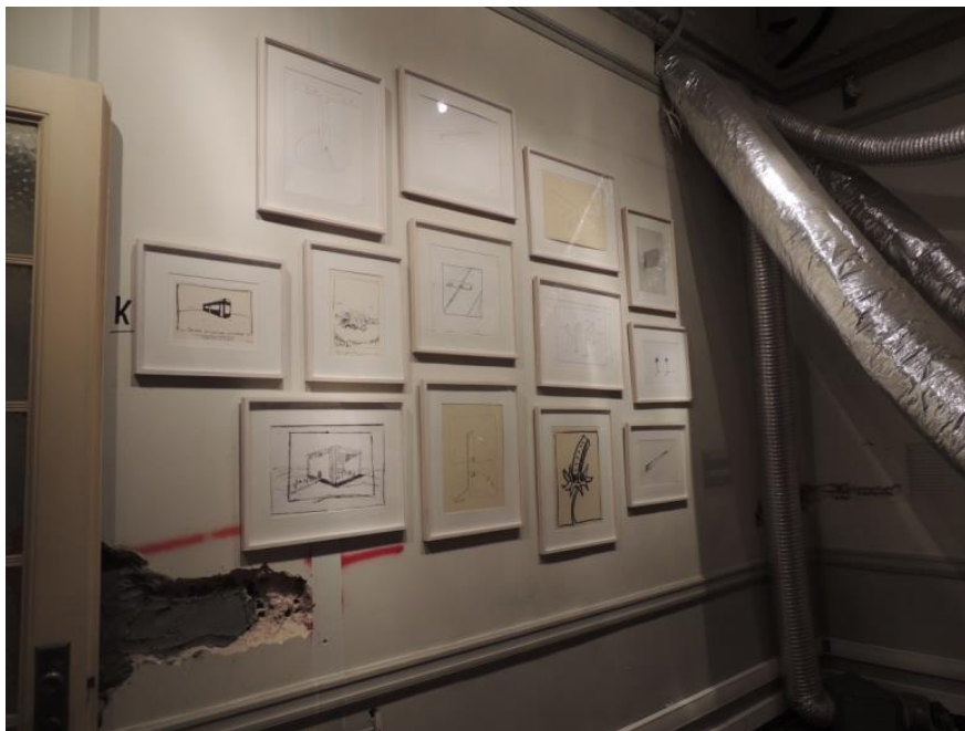
Fig 5: Cement interventions and aluminum air tubes on the inner walls at the old Stock Exchange Hall of Athens in “Agora” 2013 exhibition: M. Babousis paper artworks were lit by fluorescent tubes and there was no light radiation control. (credits: K. Stoupathis, 2013).
