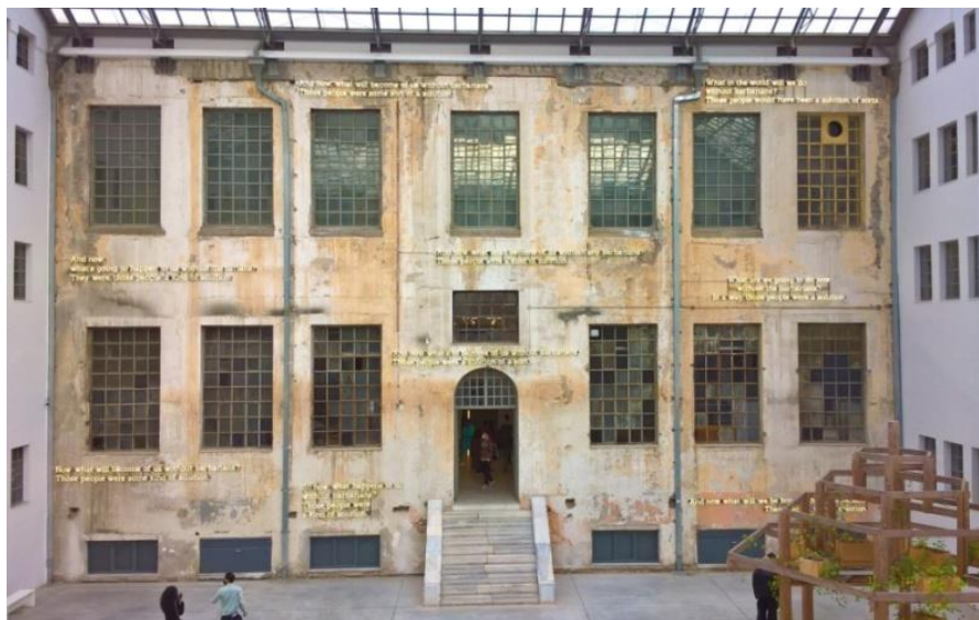
Fig 3: A site specific light installation placed onto the “Old Tobacco Factory” of Athens during “Portals” exhibition: sun-light immerses from a crystal roof (credits: K. Stoupathis, 2021).
