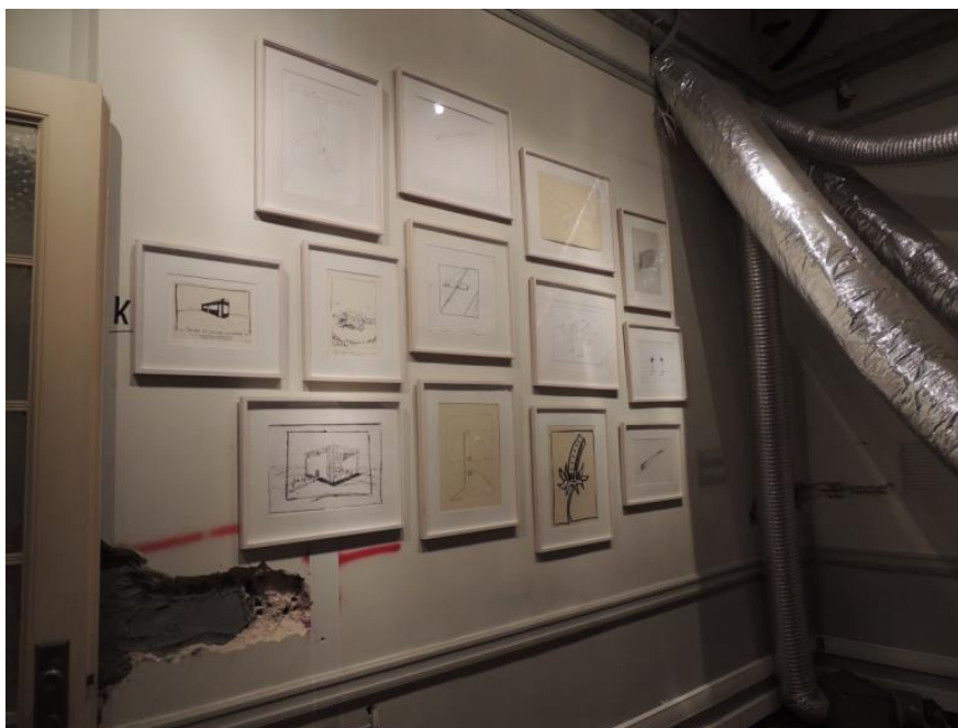
Fig 5: Cement interventions and aluminum air tubes on the inner walls at the old Stock Exchange Hall of Athens in “Agora” 2013 exhibition: M. Babousis paper artworks were lit by fluorescent tubes and there was no light radiation control. (credits: K. Stoupathis, 2013).
