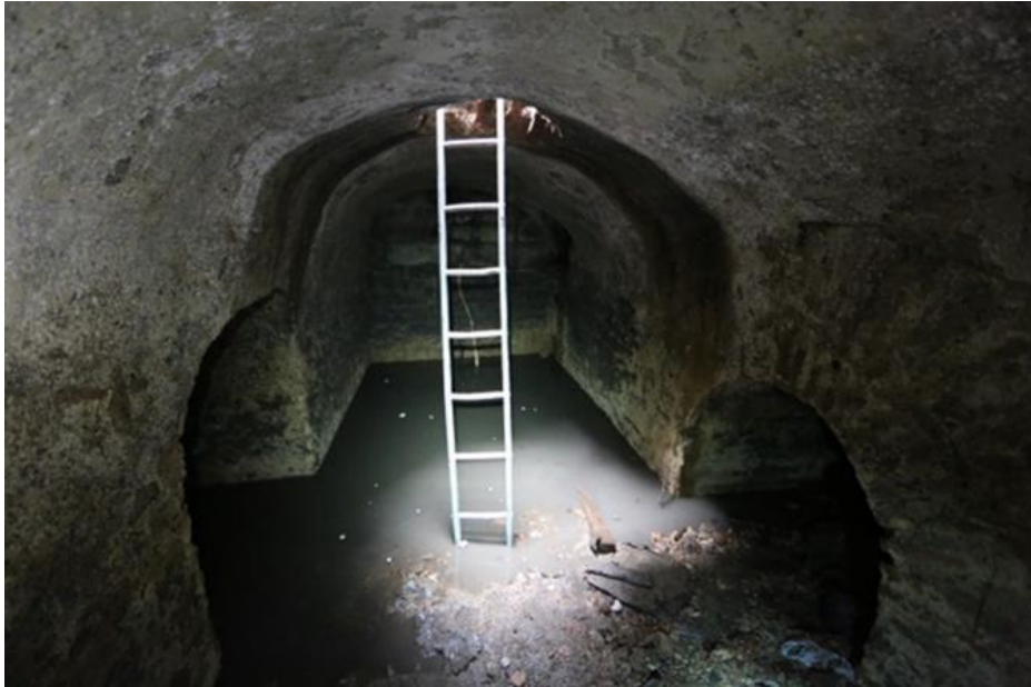
Fig. 20. View from the hypogeum in 2020 before the cleaning.
