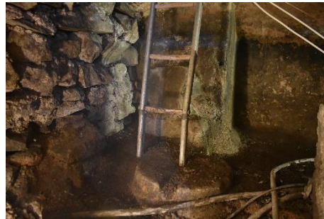
Fig. 7. The column base on the floor of the passage.
