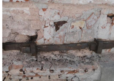
Fig. 7. Detail from the joint of the iron bracing
