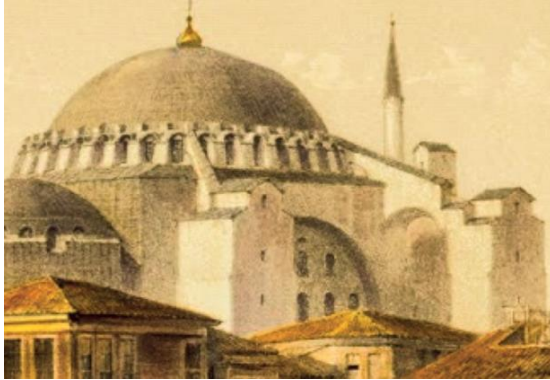
Fig. 4. Detail from Fossati's depiction before restoration
