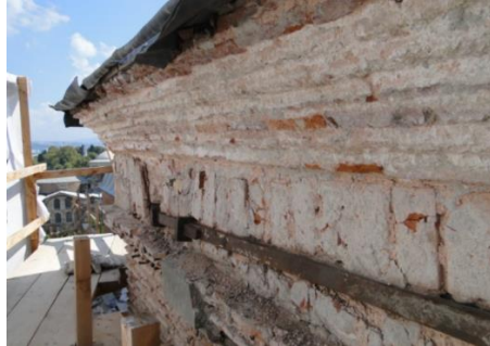
Fig. 6. Iron frame intervention under the plaster
