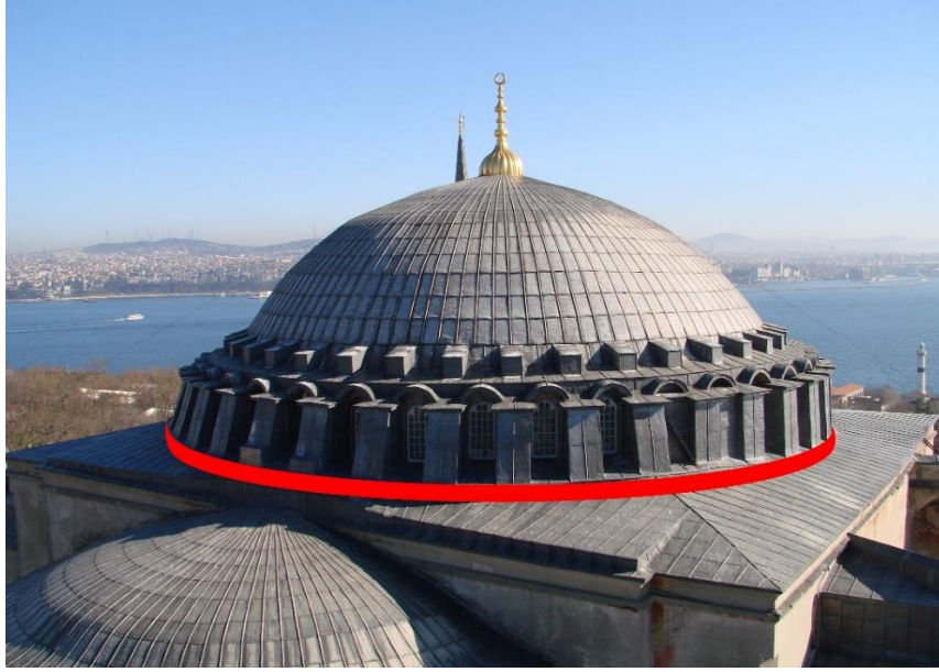
Fig. 17. Representation of the tension ring around the main dome of Hagia Sophia
