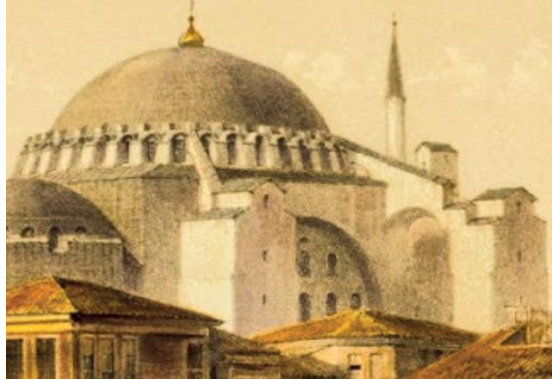
Fig. 4. Detail from Fossati's depiction before restoration
