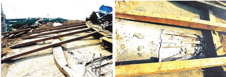
Fig. 10. Views from the partial wooden sub construction under the lead cover
