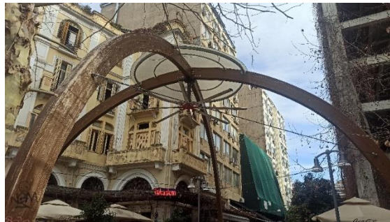
Fig. 16. Emporiou Square, view below the domed frame.
