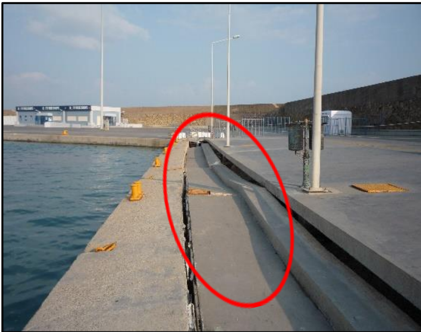
Fig. 5. Subsidence of sections of the commercial quay of Katakolo Port in 2009, circled in red. (Kiouisi et al., 2023)
