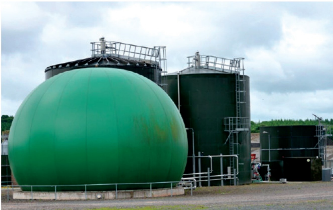
Fig. 1. Anaerobic digestors and gas holder in a farm [16]
