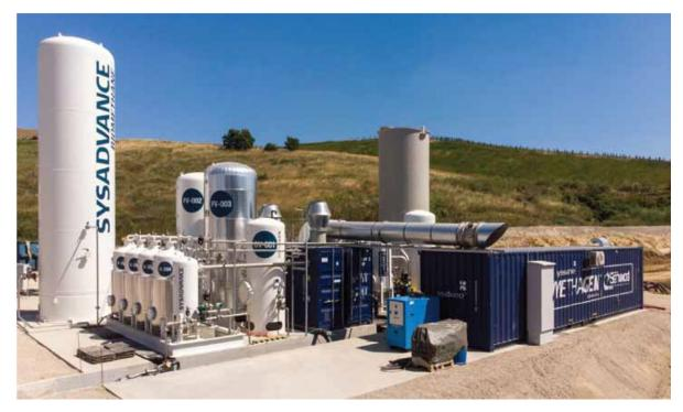
Fig. 10. METHAGEN LF system schematics for Landfill gas upgrade - SYSADVANCE
