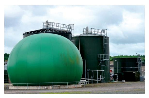
Fig. 1. Anaerobic digestors and gas holder in a farm [16]
