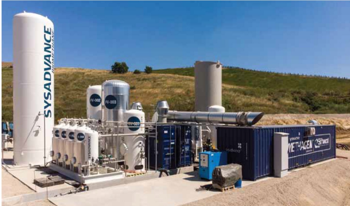
Fig. 10. METHAGEN LF system schematics for Landfill gas upgrade - SYSADVANCE
