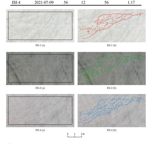
**Fig. 6.** Geospatial crack detection at the concrete area under investigation (Figure 4) for the three in-situ inspections: ISI-1 (2020-02-10), ISI-2 (2020-09-04), and ISI-4 (2021-07-09) [36] - Step 2 of Figure 2
