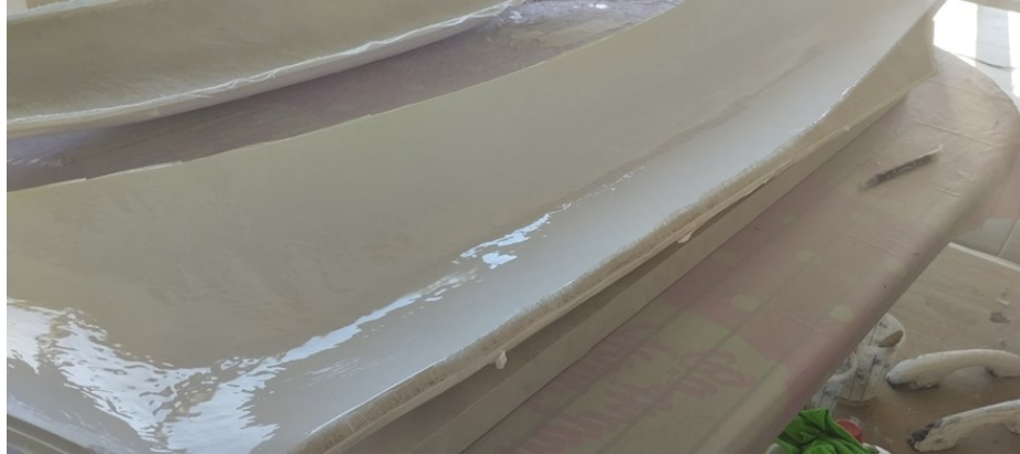
Fig. 21. The inner surface of the mold after applying Gel Coat
