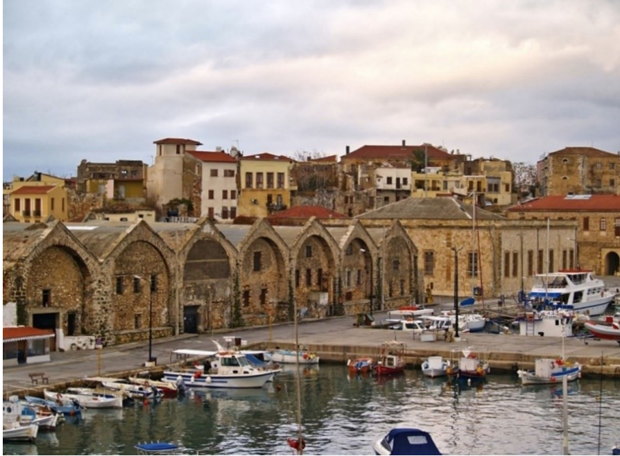
Fig. 2. The deteriorated buildings of Neoria in the center of the coastal zone, Source: Google Earth
