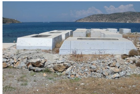
Photo 4. The large-sized cellular artificial blocks were difficult to manage, causing great dissatisfaction
