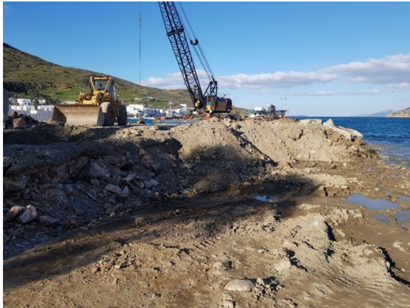
Photo 6. Heavy machinery was used to remove embankment material from the coast
