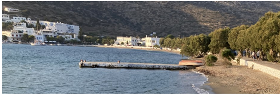
Photo 12. .....the beach is freed and naturally reshaped (2022) after the construction of the shelter
