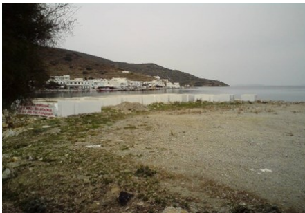
Photo 3. Embankment materials and artificial blocks deposited from the previous contract. Residents' reactions aiming to their removal were continuous, as can be seen on the protest banner
