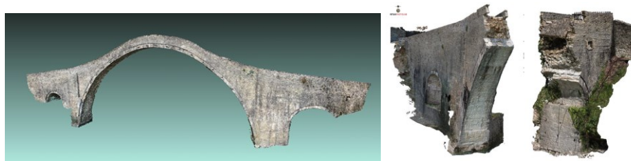
Fig. 2. Left. Orthophoto of the traditional stone bridge at Plaka, prior to its collapse, reconstructed through crowdsourced imagery. Right. 3D models of the surviving abutments of the Plaka bridge after its collapse, produced with photogrammetric techniques [32, 33]
