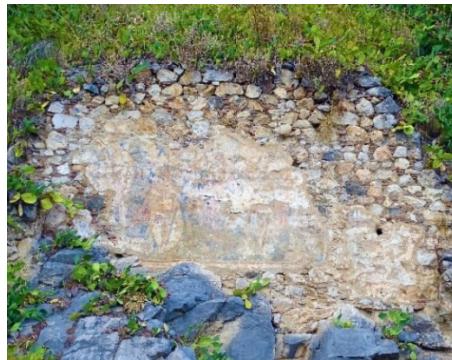
Fig. 8. Remains of a Byzantine frescoed chapel on the ring road of the castle [36]
