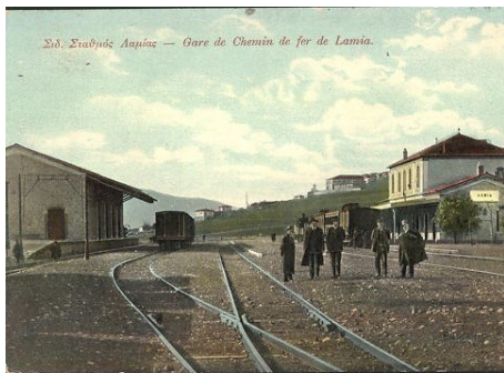
Fig. 19. The railway station of Lamia (1900-1910) [28]
