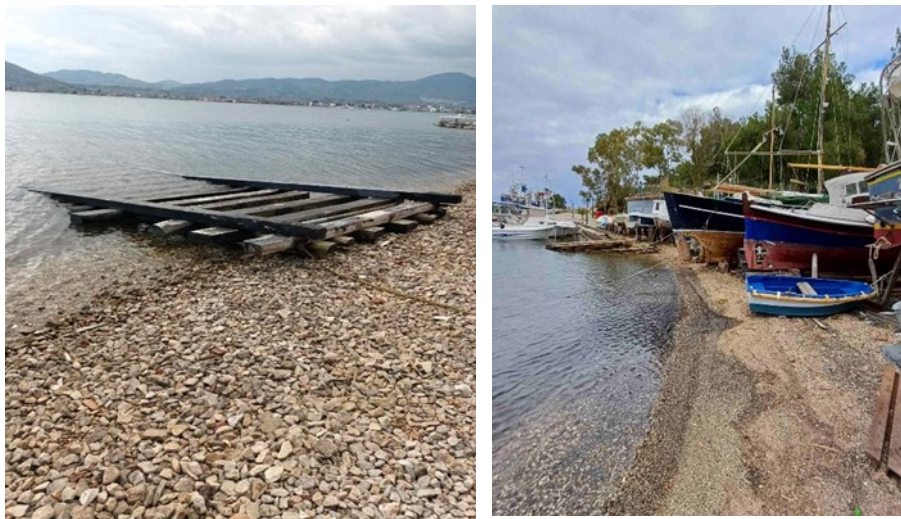
Fig. 6. Typical shape of sxara (left) which serves for launching and berthing (right) procedures
