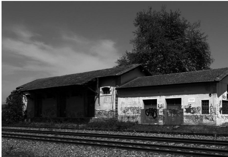
Fig. 11. Exterior view of the building's current condition [25].
