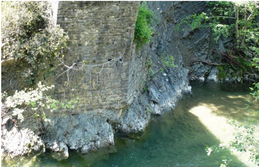
Fig. 5. Revelation of the foundation
