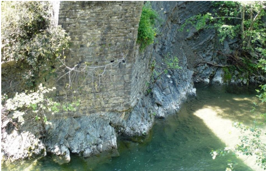
Fig. 5. Revelation of the foundation
