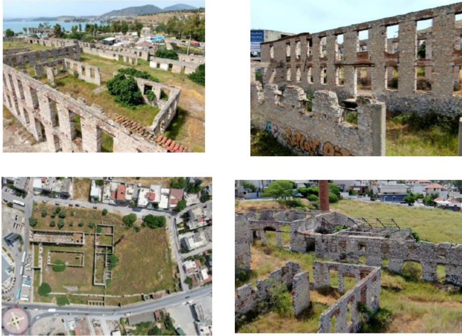
Fig. 2. Exterior views of the complex's current condition.
