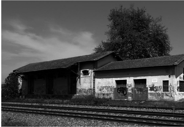
Fig. 11. Exterior view of the building's current condition [25].
