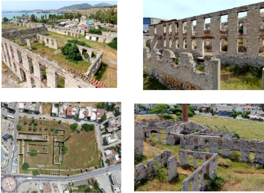
Fig. 2. Exterior views of the complex's current condition.
