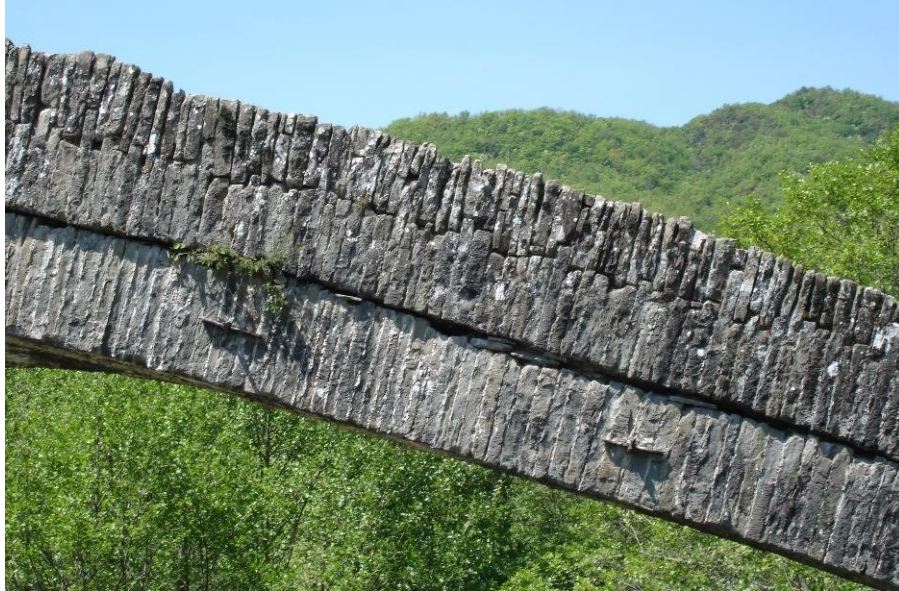
Fig. 4. Loss of contact between the two rings
