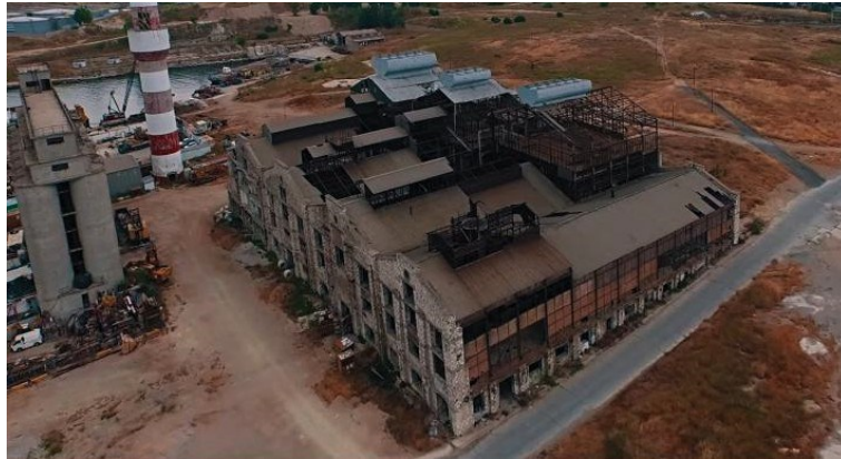
Fig. 14. Aerial view of the building's current condition [26].
