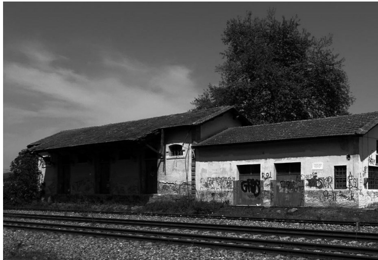
Fig. 11. Exterior view of the building's current condition [25].
