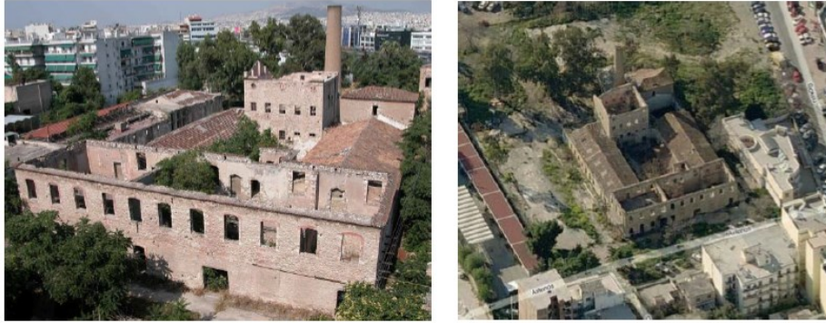
Fig. 5. Exterior views of the complex's current condition.
