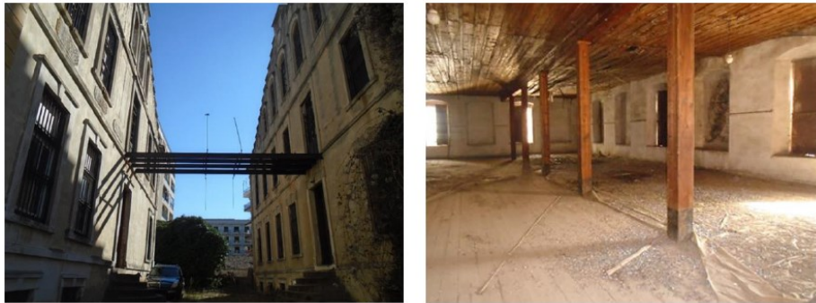
Fig. 8. Exterior and interior views of current condition.
