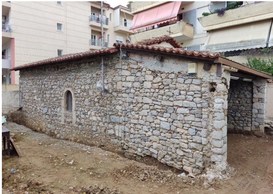
Fig. 2. North–West view of the church. Removal of plaster on the exterior masonry. Excavation of the northern part of the surrounding area. (24/9/2022)
