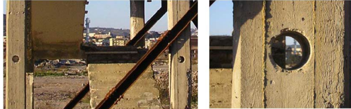
Fig. 10. Extraction of cylindrical cores from module n.6.
