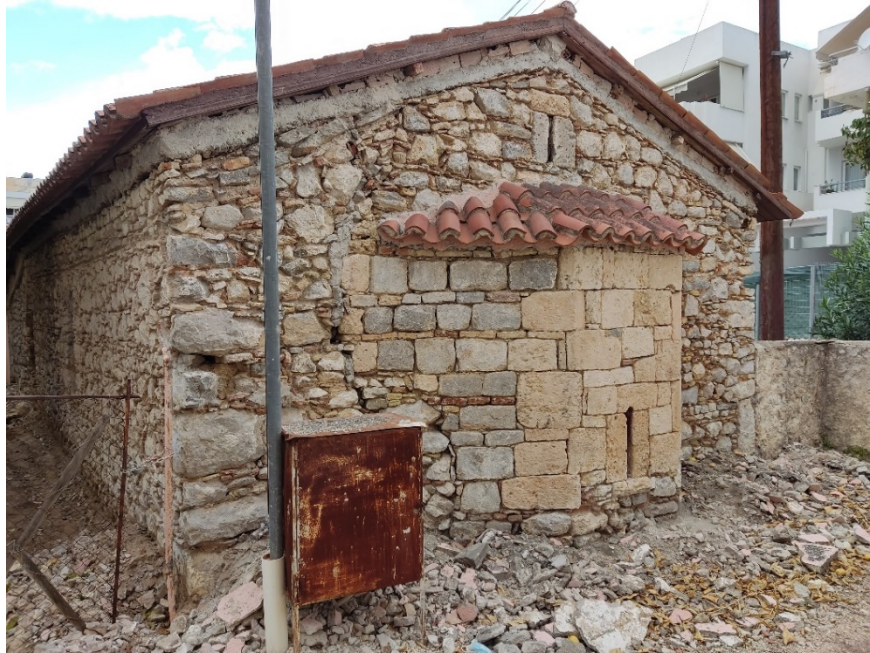
Fig. 3. South–East view of the church. Removal of plaster on the exterior masonry. (24/9/2022)
