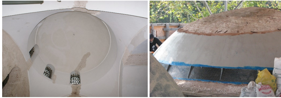
Fig. 16. View from the crack under the dome and CFRP intervention above the dome.
