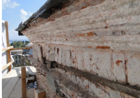
Fig. 6. Iron frame intervention under the plaster
