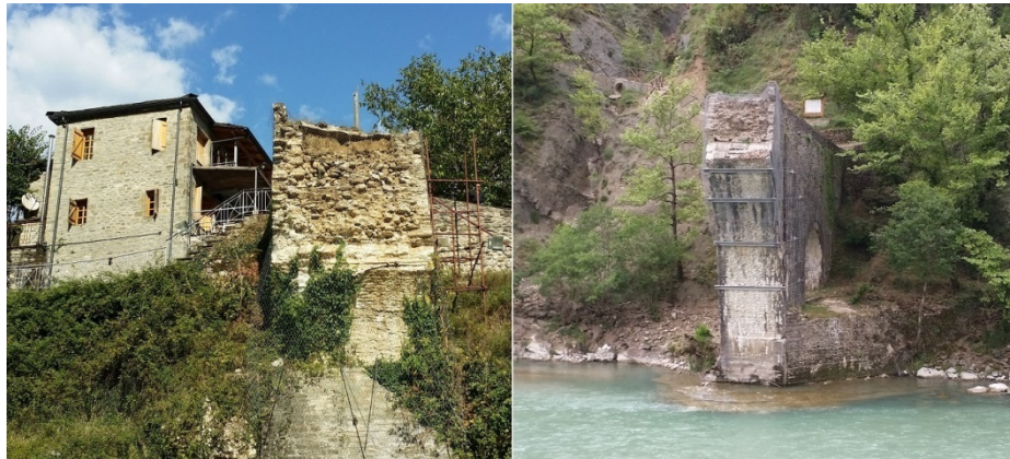
Fig. 6. Surviving sections of Plaka Bridge, September 2018. Left: part of east abutment and the Customs building. Right: West abutment and piers body.
