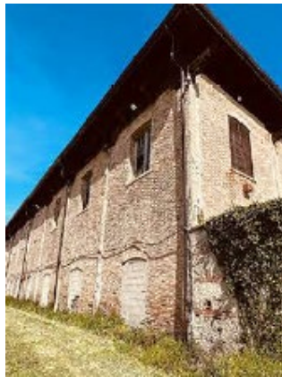
Fig. 10. Closure of the opening at ground floor
