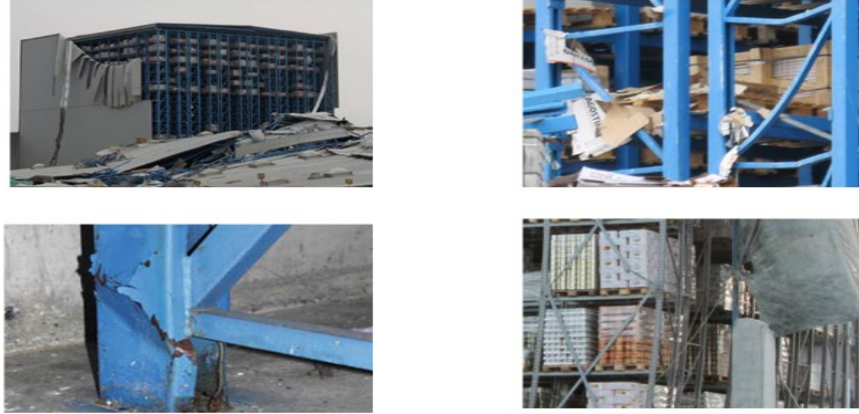
Fig. 10. Failure of steel racks making part, or not of the lateral load resisting system, Emilia earthquake, 2012 [70]
